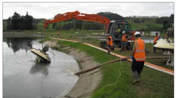
TE KUITI WASTEWATER TREATMENT PLANT UPGRADE
